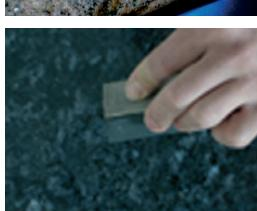
Carefully remove excess material with AKELUX Planer. For limestone, we recommend the use of cuttlebone. This step is not necessary when using a surface structure stamp.
