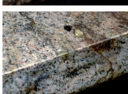
Mix AKELUX Filler transparent liquid with different coloured AKELUX Fillers (max. 50% colour portion) and adapt as closely as possible to the object colour. If necessary, fill with AKELUX Structure.
