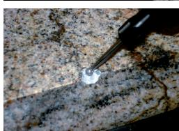
Mill out the damaged area and remove all loose parts and dust. Milling can be done manually or mechanically.
