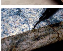
Mask the damaged area at the edge with transparent tape. Then apply AKELUX Filler transparent liquid or AKELUX Filler transparent gel crystal for the first filling. Cover with AKELUX Transparent Film or, in the case of textured surfaces, with a surface structure stamp\*\* and harden 60 s/cm<sup>2</sup> with AKELUX LED Light Emitter\*.
