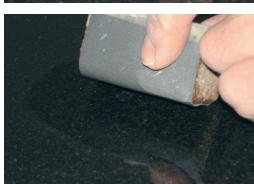
Place AKELUX Silicone Abrasive Cloth on the AKELUX Grinding/Polishing Block and wet grind the damaged area in the sequence 2400-3200-4000. This step is not necessary when using a surface structure stamp.
