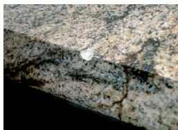
Break-off or chipping of an edge in natural or artificial stone (s. a. marble, granite, quartz) as well as ceramics (e.g. kitchen countertop, window sill, bathroom, stair tread).
