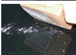
Carefully remove excess material with AKELUX Planer. For limestone, we recommend the use of cuttlebone. This step is not necessary when using a surface structure stamp.
